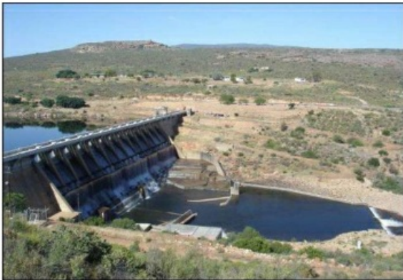
Clanwilliam Dam prior to raising
